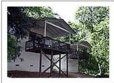
Large One Bedroom - Exterior
